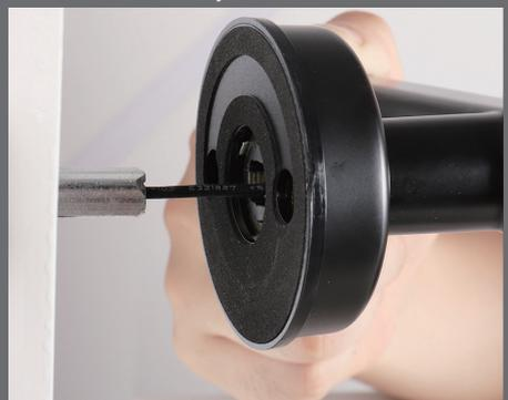
Put one end of the power cord through the center hole of the outside handle.
