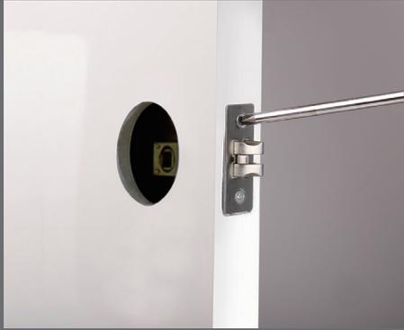
Push the latch into the Latch hole & install the two M4 x 18 Latch screws
