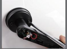
Align the square spindle & install long handle screws to mount the inside handle to the outside handle
